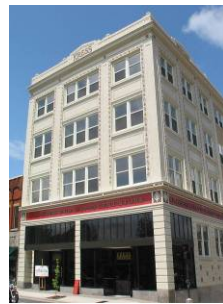
The rehabilitated Kress building.
