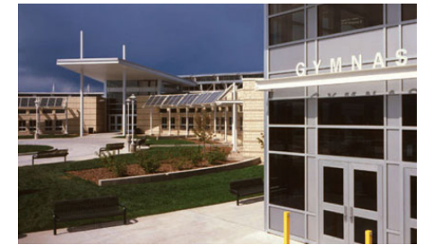
Fossil Ridge High School in Fort Collins Colorado was built to Poudre School District's Sustainable Guidelines
