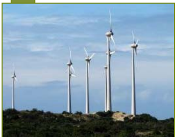
Wind energy conversion system
