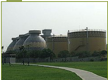
Sewage treatment plant
