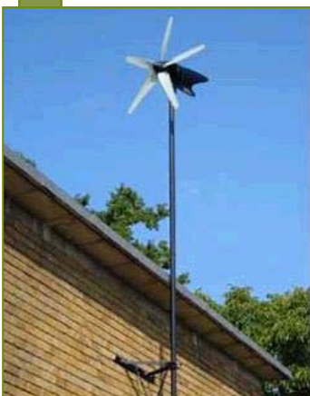
Wind turbine (building mounted)
