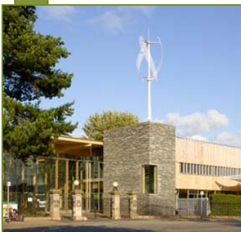
Building mounted wind turbine
