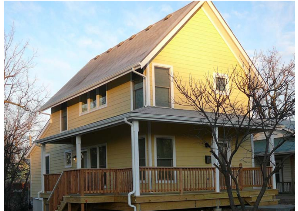
This Habitat for Humanity home in Kansas City includes optimized solar orientation to take advantage of southern exposure, high efficiency plumbing fixtures, a geothermal heat pump, and salvaged and recycled materials.
