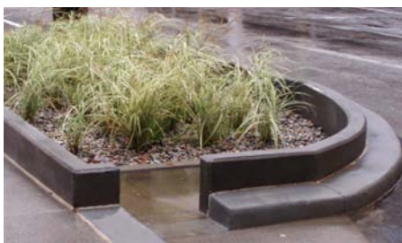
This rain garden captures runoff from the street and uses it to irrigate the plantings.
