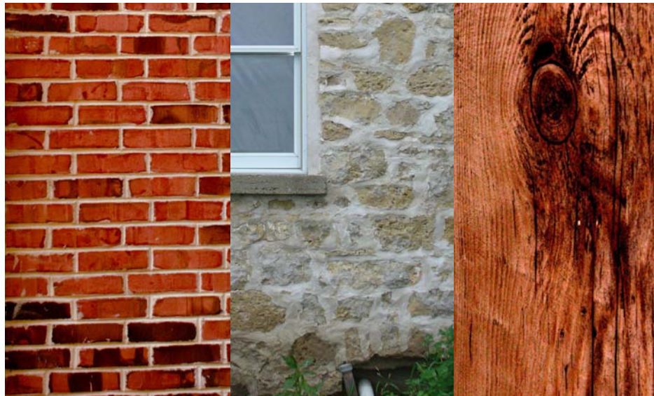
(Top) Some homes in Greensburg are choosing to use SIP panels to better insulate their homes. (Bottom) Some common durable building materials include brick, limestone and wood, when used appropriately and with quality detailing and design. Concrete and steel are other durable materials often incorporated into building projects.
