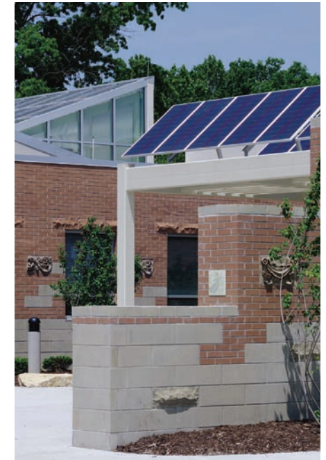
Solar panels can be added to further decrease energy use.
