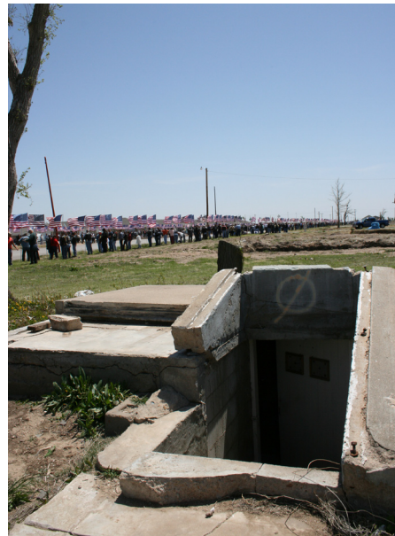
A storm cellar in Greensburg likely protected citizens through many storm events.
