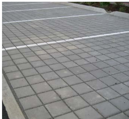
Creative stormwater capture (top), bioswales (middle), and pervious parking (bottom) are all techniques for integrated stormwater management.
