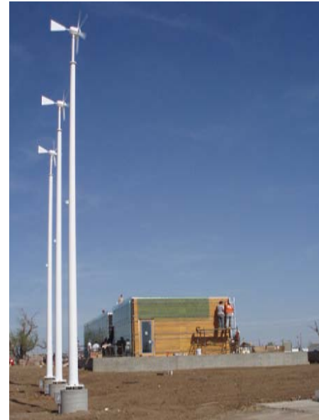
These small turbines installed at the 5-4-7 Art Center in Greensburg enhance the building with renewable on-site energy and are quiet to prevent disturbing the neighbors.
