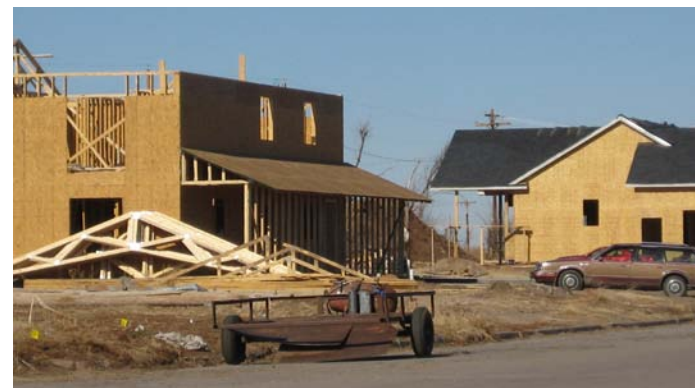
Home construction in Greensburg in January 2008.
