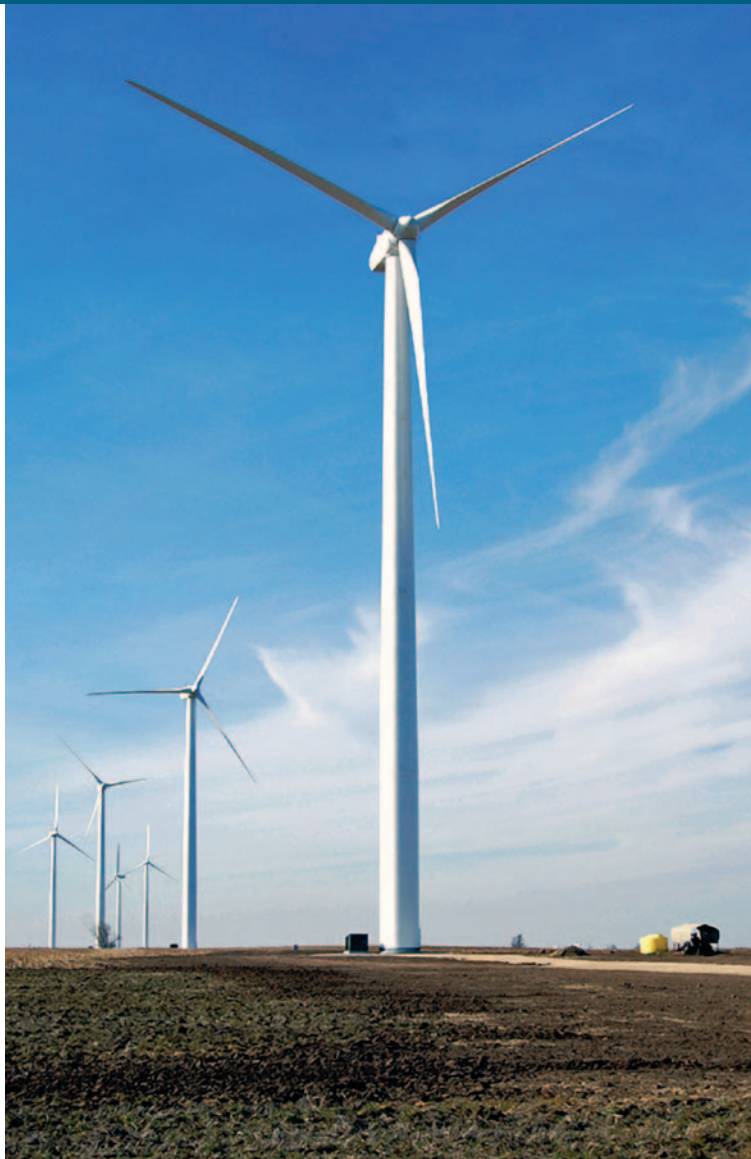
The Greensburg Wind Plant in Kansas, comprising ten 1.25-megawatt wind turbines, supplies enough energy to power every house, business, and municipal building in Greensburg.
