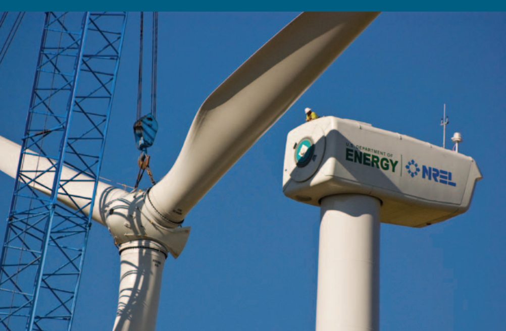
Blue skies and calm conditions contributed to a smooth installation of the DOE 1.5 megawatt wind turbine at the National Wind Technology Center.
