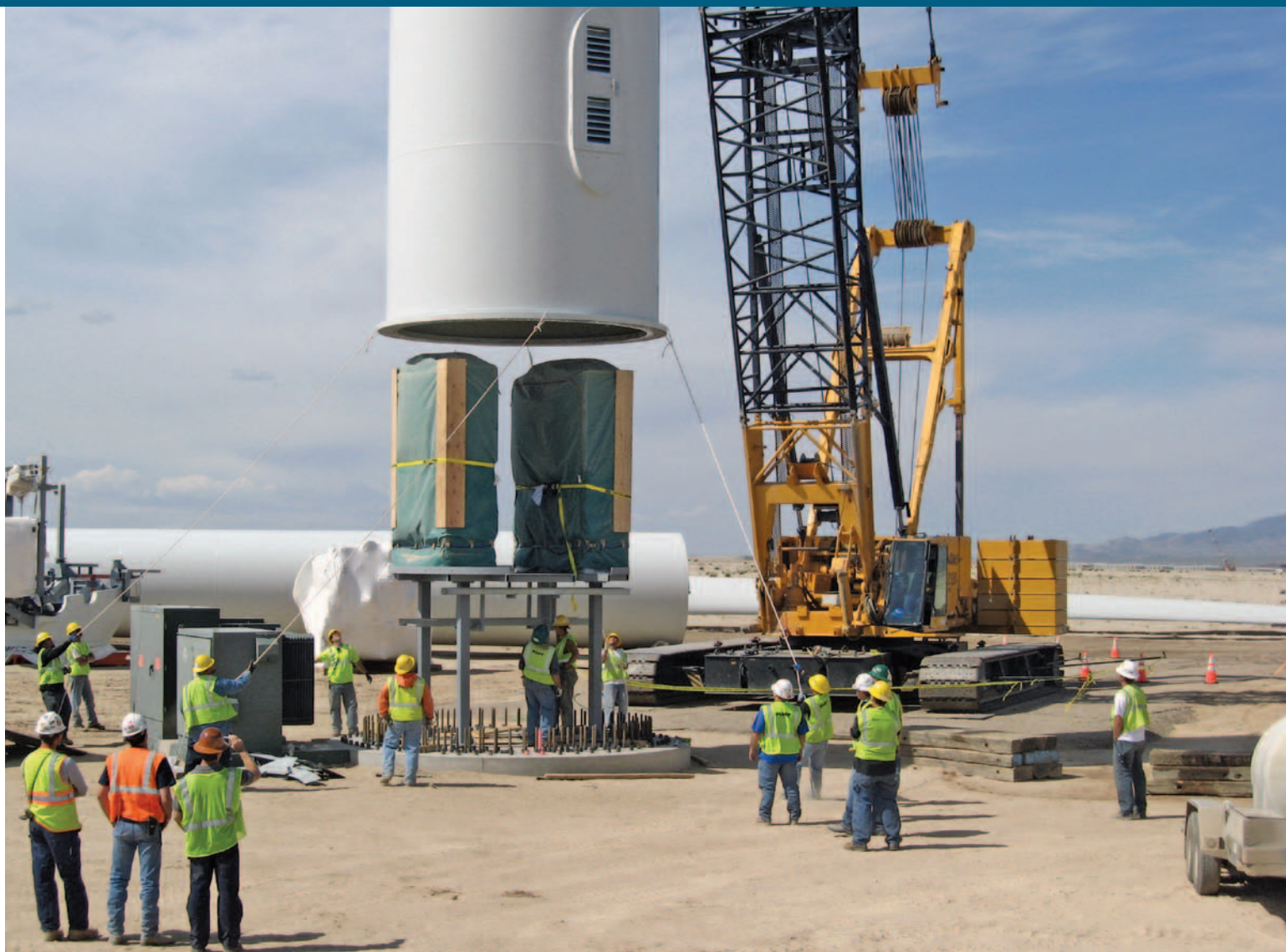
Construction workers in Milford, Utah, lower the first section of a tower for a multimegawatt wind turbine.
