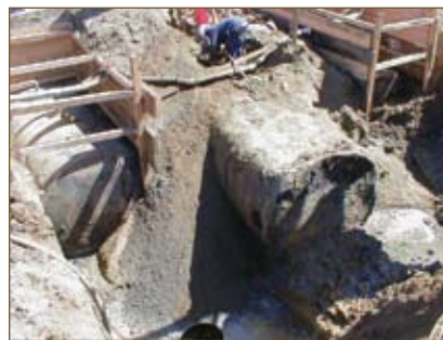
Workers unearth large underground storage tanks
