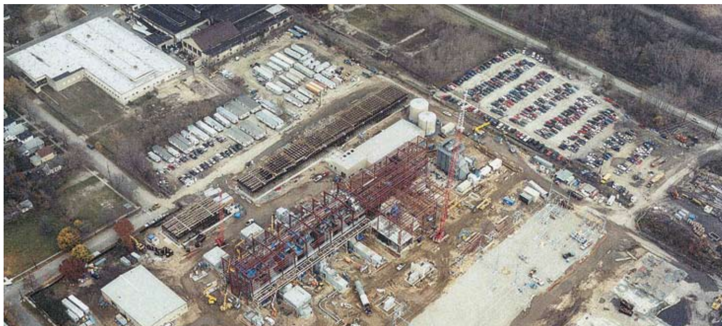
Construction activities at the Kinder Morgan Jackson Power Plant
