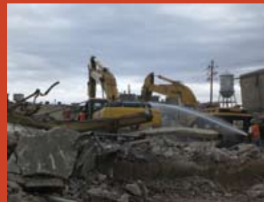
Demolition at Gates Rubber Plant, Denver, CO
