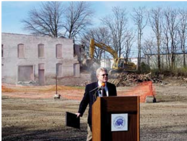
Demolition of the F.C. Cline Building
