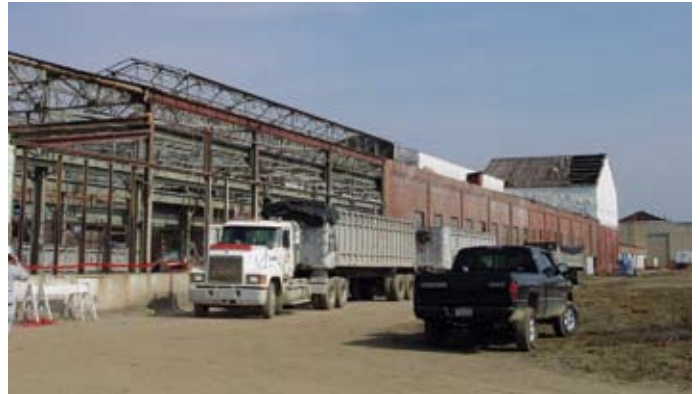
Construction activities at the former PPG Factory
