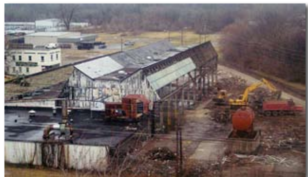
Prime Battery site before demolition
