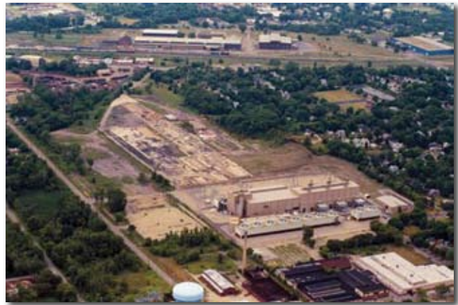
Aerial view of the redeveloped Goodyear property
