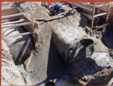
Underground Storage Tank removal
