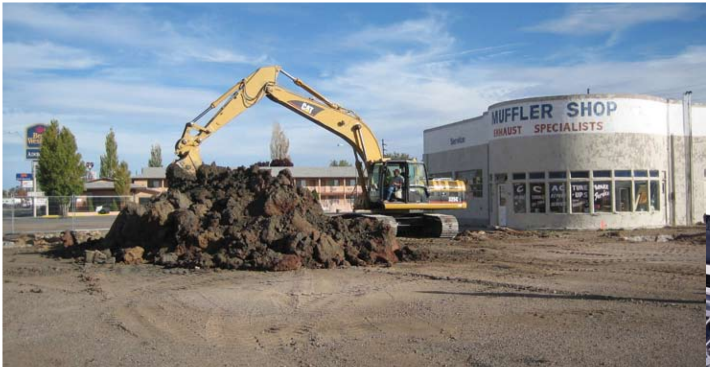
Digging up an UST outside a muffler shop along Route 66
