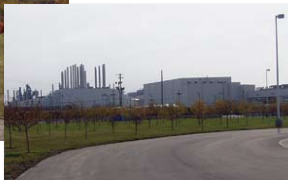
Rows of trees greet visitors to the truck plant at the Ford Rouge site
