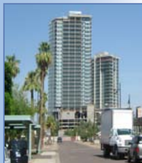
Centerpoint Condominiums in Tempe. Courtesy of Philip Armorosi, Arizona Department of Environmental Quality
