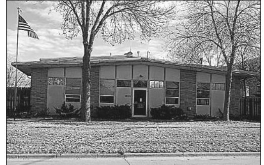
St. Anthony Public Works Department Facility
