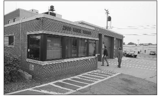
St. Anthony Fire Department Facility
