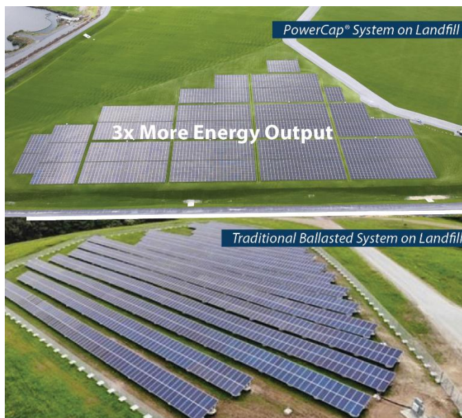
A visual guide to the difference between the PowerCap® system and a traditional ballasted system. Photo by TVA.
