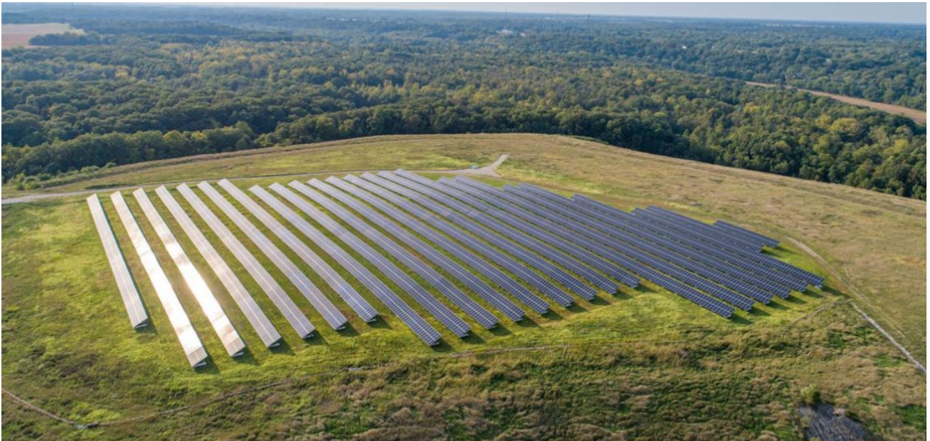
Array of the solar deployment project in Danville, Illinois.
