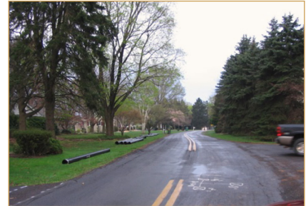
Preparations are made to extend public water lines to properties.
