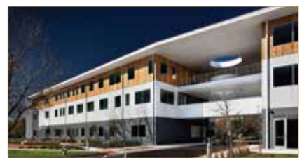
An AEGB-rated 5-star building
