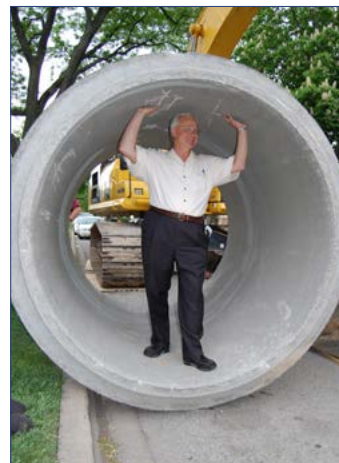
Ensuring a stable foundation for the stormwater system. (Photo credit: Tom Robb, Niles Journal, Journal & Topics Newspapers)
