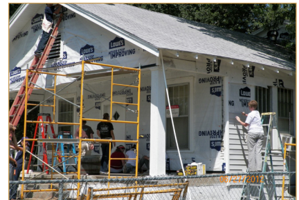
Volunteers with World Changers install siding on a Fort Smith residence.
