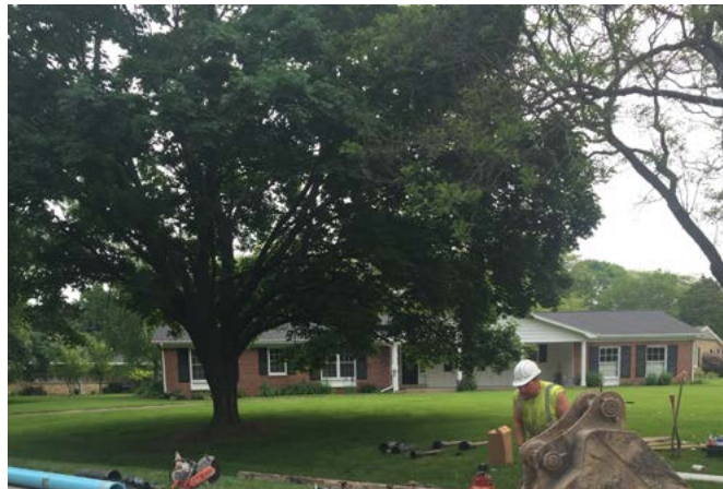
Converting to a municipal water system.
