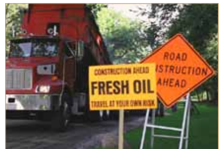
A joint roadway resurfacing project was bid via the MPI.
