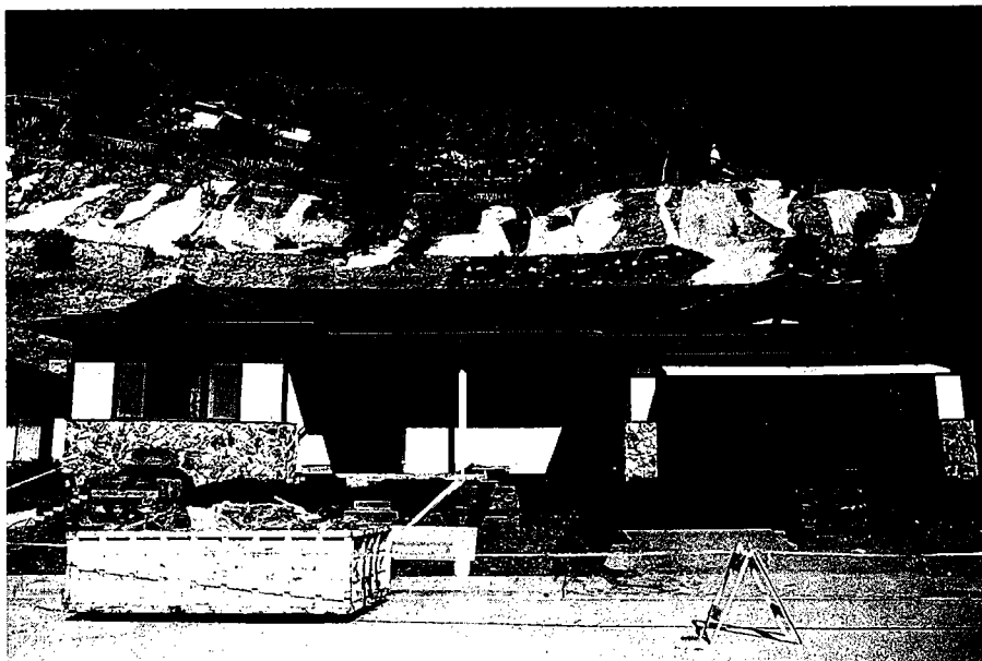
Houses like this one that were in the path of the landslide in San Leandro, California, were moved forward to the edge of the curb and set on railroad ties.
