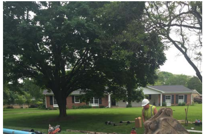
Converting to a municipal water system.
