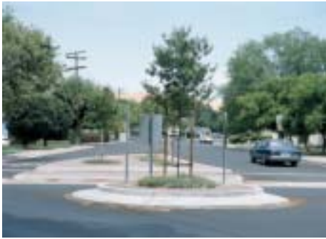
The new traffic circle at Landana Dr. and Mulberry Dr. slows speeding cars.
