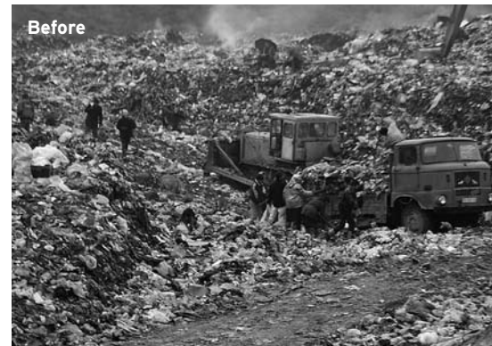
Sharra Landfill before 2005 and after in 2007
