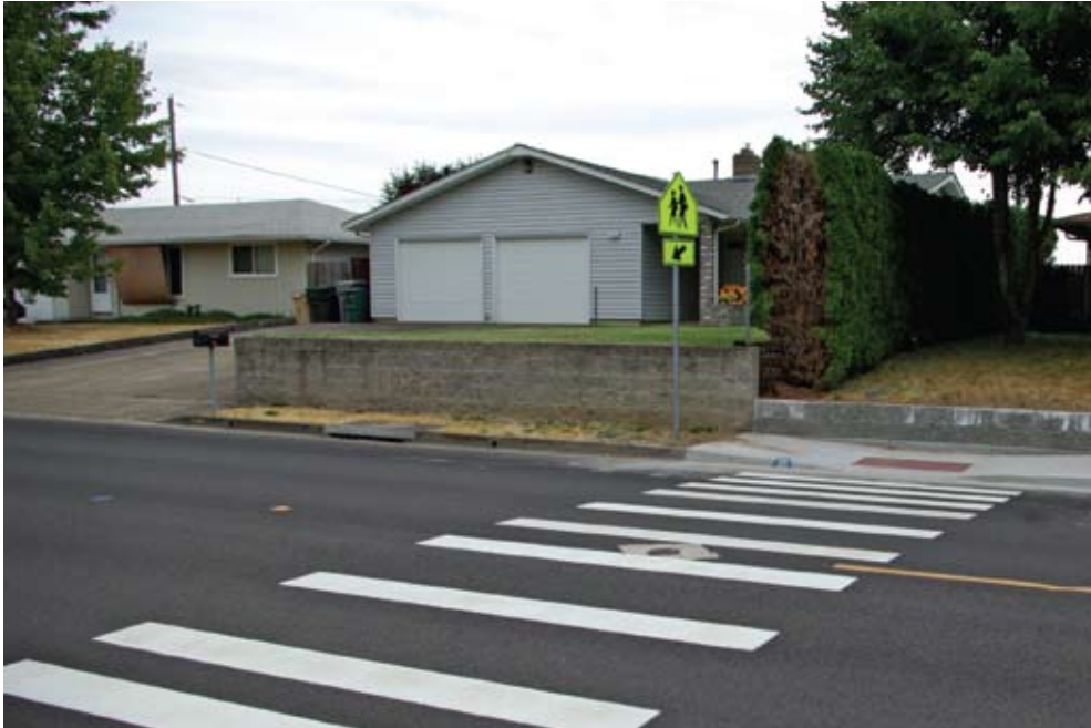
A new pedestrian crosswalk installed in South Albany near Oak Elementary School to make it safer for students to walk to school.
