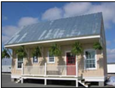
The Katrina Cottage prototype, designed by Marianne Cusato, features two small bedrooms with an additional sleeping loft, full bathroom, kitchenette, and living room. It is more wind resistant and sturdier than a FEMA trailer and costs $10,000 less. Source: http://www.slate.com/id/2138981/
