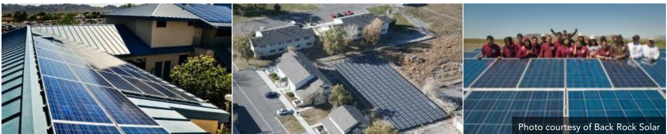
Black Rock Solar. From left to right: College of Southern Nevada, Pershing General Hospital, Pyramid Lake High School.
