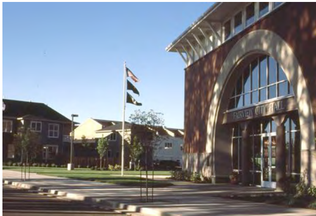
Fairview Village City Hall and nearby housing.
