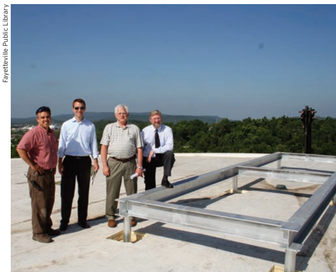
City, library, and community partners at the solar test-bed installation on top of the Fayetteville Public Library.
