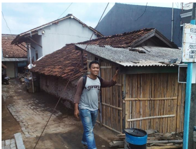
Figure 8. Land subsidence in Tambak Rejo
