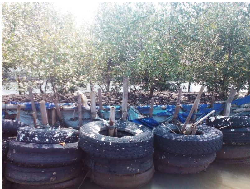
Figure 6. Mud-filled car tires for wave breakers and mangrove protection
