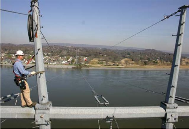
An EPB employee works on fiber optic cables extending over the Tennessee River. Photo courtesy of EPB.
